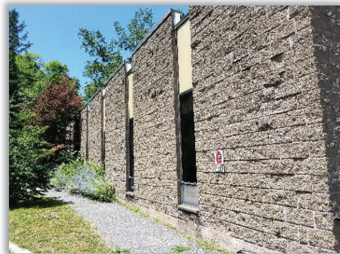
Figure 2.15: The Putnam Family & Community Services building located at 1808 Route 6
