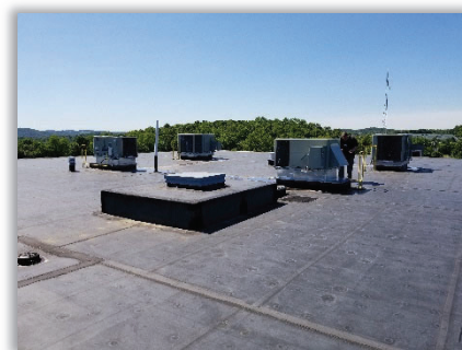
Figure E24.3: Existing flat roof at the Kern Building
