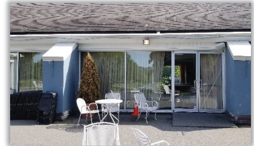
Figure E17.1: Existing aluminum windows and doors at the Golf Clubhouse
