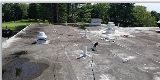
Figure E24.1: Existing roof at the Golf Clubhouse
