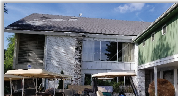
Figure E23.1: Existing wood and brick exterior of Golf Clubhouse.
