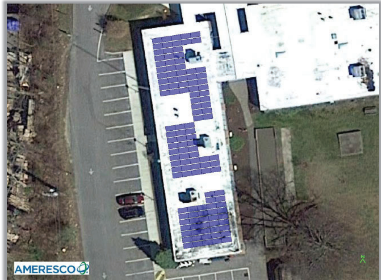
Figure E18.4: Site diagram/illustration that includes location/design of array, and proposed capacity (45.3 kWdc)
