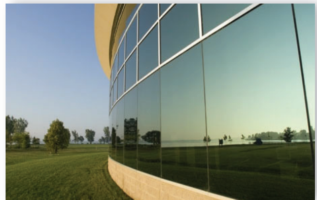
Figure CNR21.1: An example of commercial size windows that have had window film installed.
