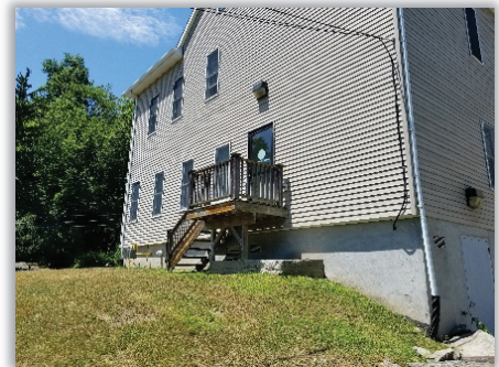
Figure 2.22: The Putnam Family & Community Services building located at 1816 Route 6
