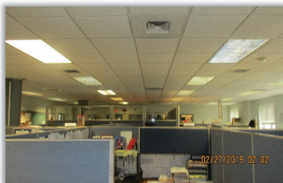
Figure E1.1: This project will improve aesthetics and provide substantial energy savings.
