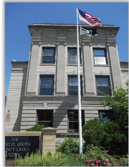
Figure 2.3: The Bruen County Office Building
