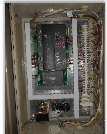
Figure E3.4: Current Andover Controls
