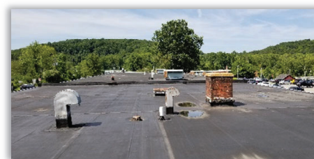
Figure E24.2: Existing roof at the Smith Building 3
