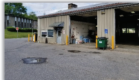
Figure 2.18: The Highway Department – Building 3 Dispatch/Garage
