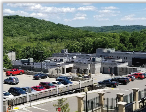
Figure 2.1: Putnam Sheriff's Department and Correctional Facility
