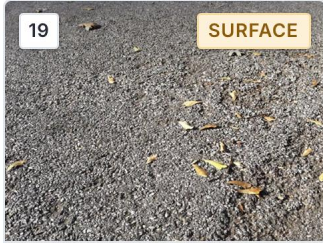
Raveling Aggregate loss · SF
