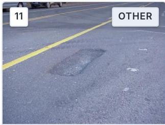
Patching & Utility Cuts Repair · SF
